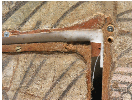
Figure 19. Closed-cell cross-linked polyolefin foam T-Cell® EVA was inserted behind thinner panels to bring these into plane with a thicker, neighbouring panel. Photo: Courtesy of the Royal Ontario Museum, ©ROM.
