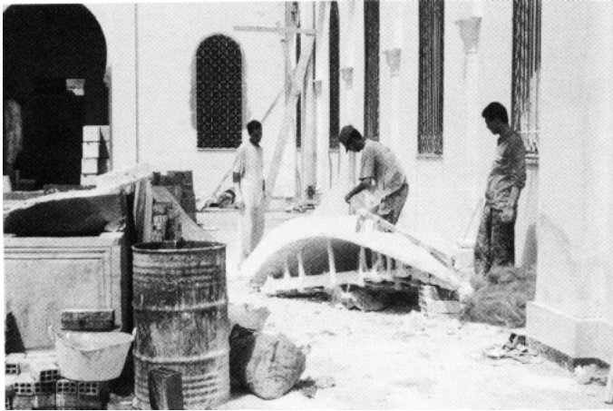
Figure 2. Construction of vaulted ceiling sections according to traditional Tunisian construction methods.
