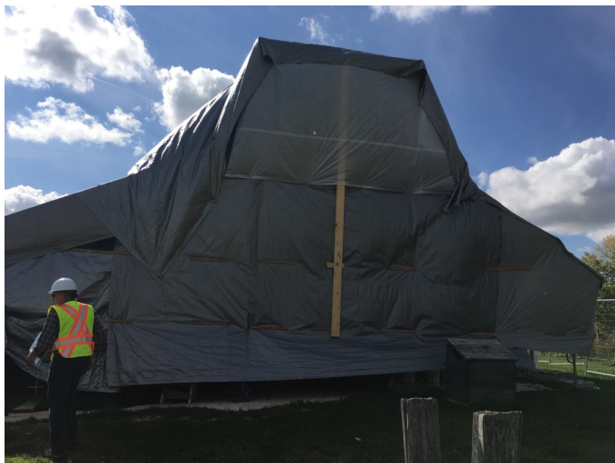
The Farm Managers House tented so that temperature-controlled painting, white washing, and window repair can occur.
